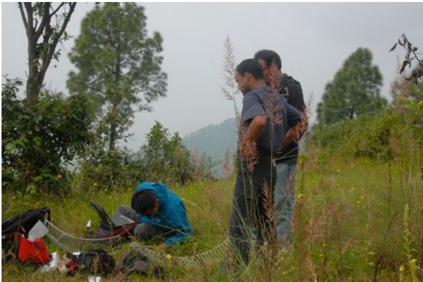
Figure CSD 5: Preparing for relay installation, Kumaon Network
