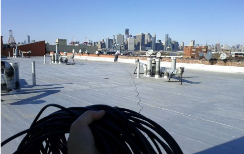
Figure CsOTI 5: Running cable to install a node on the roof of an apartment building north of Coffey Park.
